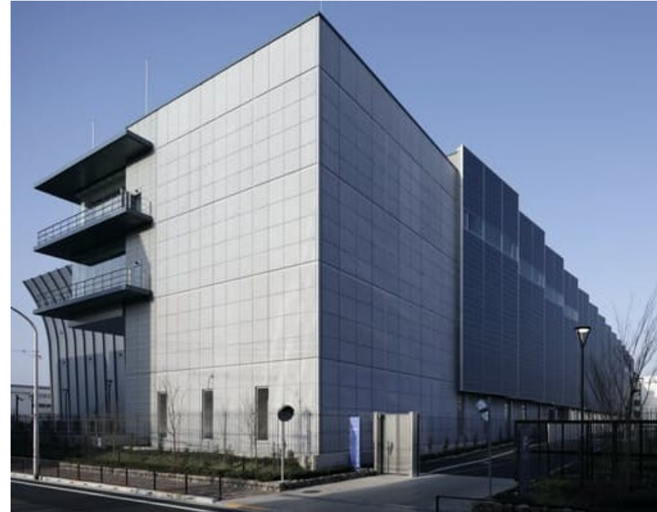
Energy efficiency of data centers is being improved
